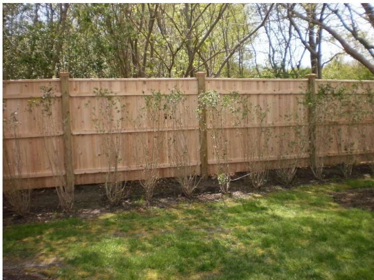
Ambassador with moulded cap dowed into 5x5 posts with post caps
