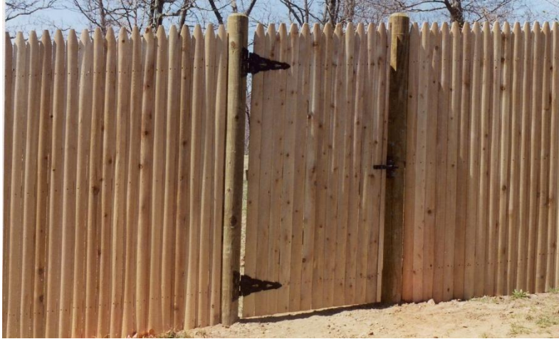
Traditional stockade dowelled into round pressure treated posts
