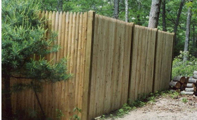
7' tall stockade dowelled into 5x5 pressure treated posts
