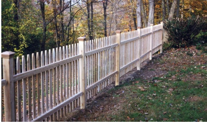
Spaced stockade dowelled into 4x4 posts with post caps
