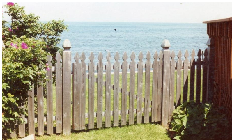
Spaced Williamsburg fence dowelled into 5x5 cedar posts
