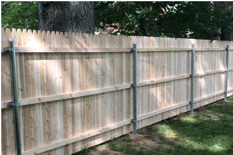
Stockade attached to commercial grade SS-20 steel posts
