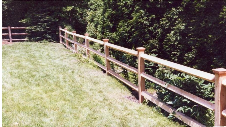
Three high Estate rail 5x5 posts & 4x4 rails
