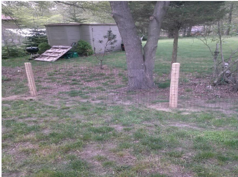
Welded wire attached to round wood posts
