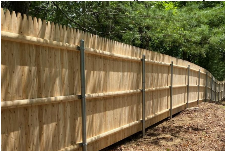
Stockade attached to commercial grade SS-20 steel posts with moulded back rails
