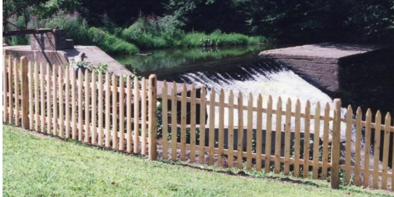
Spaced stockade dowed into round cedar posts
