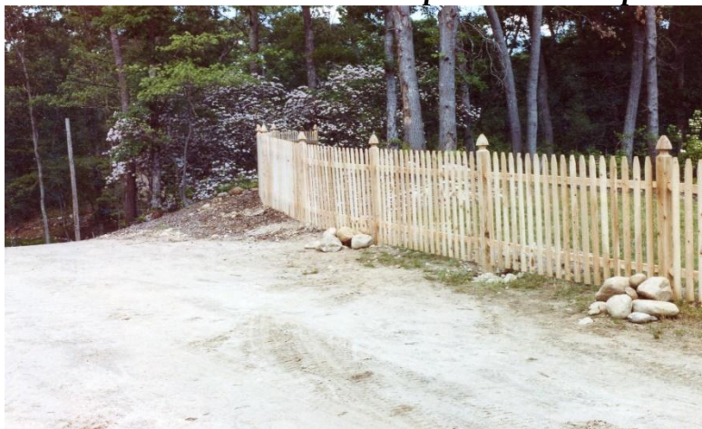
Spaced stockade dowed into 4x4 gothic posts
