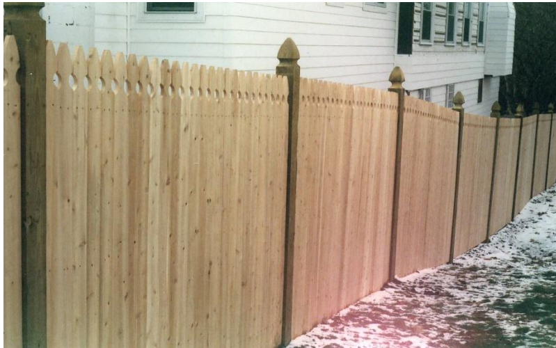
Solid board Williamsburg dowelled into 5x5 gothic pressure treated posts - Outside view
