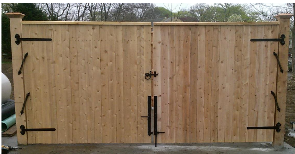
Double gate with snug cottage hardware and gate springs
