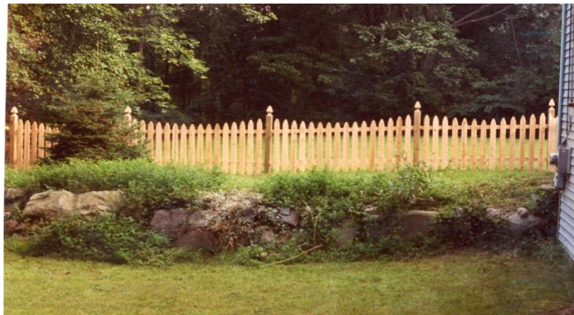
Gothic spaced board fence dowelled into 4x4 gothic posts
