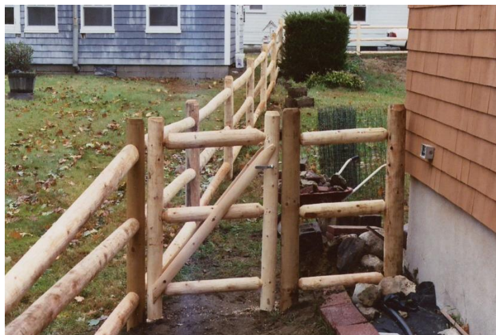
Round rail single fence gate three high
