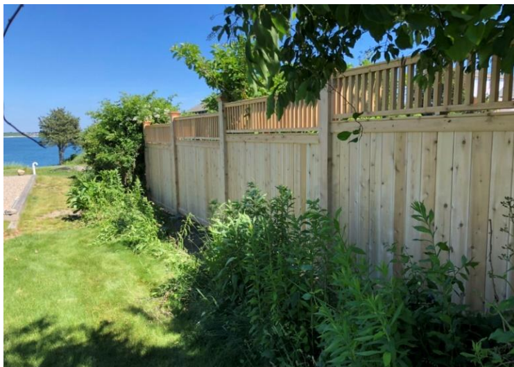
Tongue and groove with closed Mt Vernon topper – Outside view
