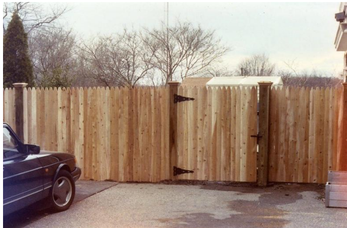
6' stockade dowelled into 5x5 pressure treated posts with post caps
