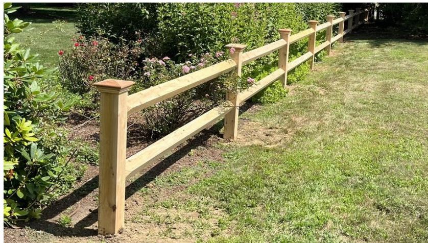
Two high Estate rail 5x5 posts & 4x4 rails
