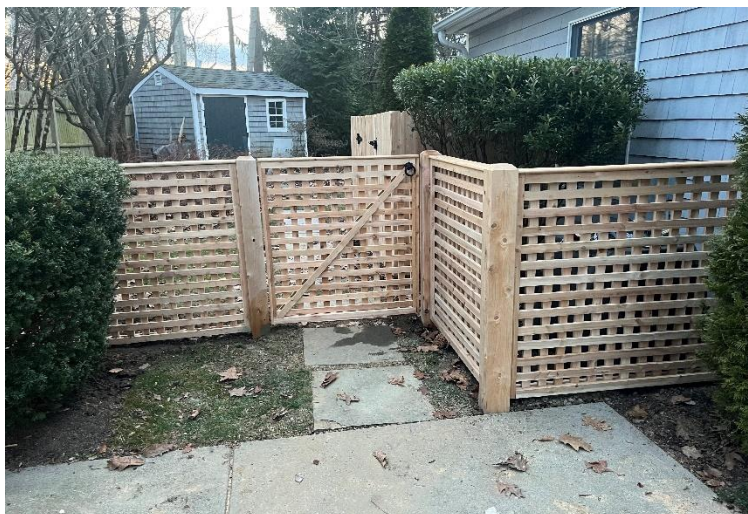
4' high lattice on 5x5 chamfered posts
