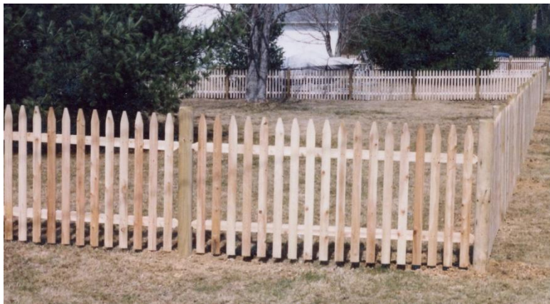
Spaced stockade dowed into round pressure treated posts
