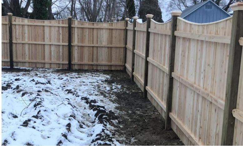
Estate style 6' board screen dowelled into 5x5 pressure treated posts (Inside view)
