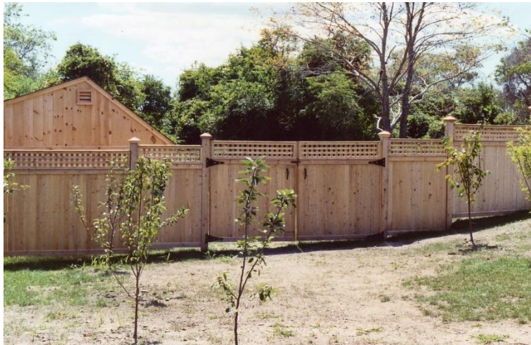
Fence stepping up hill with double gate
