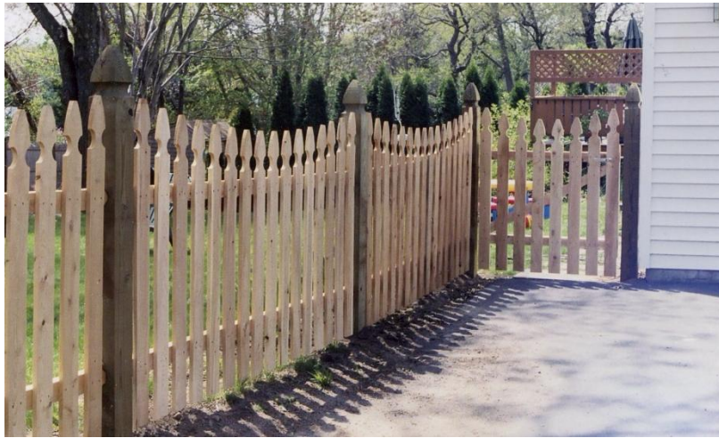
Spaced Williamsburg dowelled into 5x5 pressure treated posts
